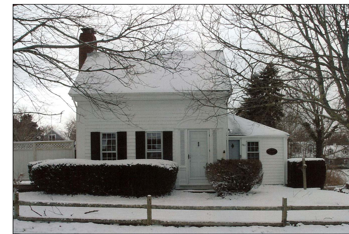
Architect & Contractor: Polhemus Savery DaSilva, Chatham, MA
