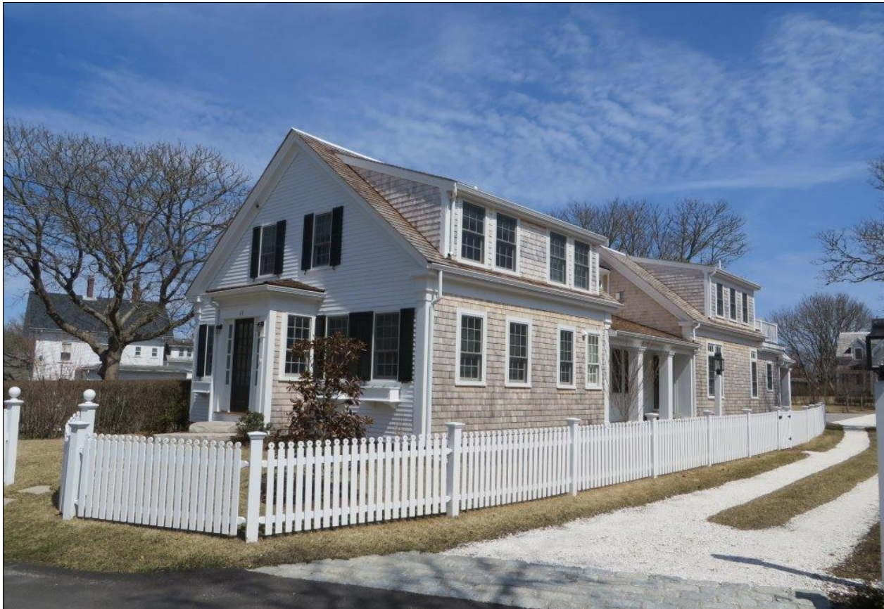
11 Shattuck Place • The David Elmer Howes House Owner: Robert and Margaret MacDonald
